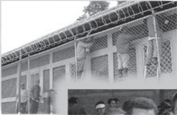
PAINTING THE NEW CLINIC: INAUGURATION JUNE 28, 2005
